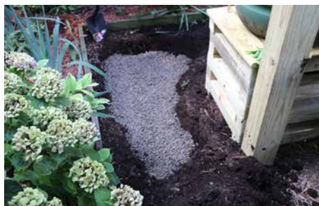
To help prevent any possible flooding from the downspout on this system, a small rain garden was installed next to the overflow from the rain barrels. This small 4x5' area—excavated and filled with gravel, landscape fabric, plants, and stepping stones—will provide an overflow area for any excess water entering the system.
