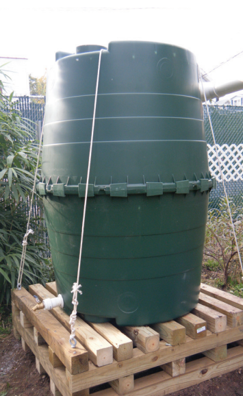
This tank is anchored to a wooden base with eyebolts and rope. A spigot is connected by a bulkhead fitting.
