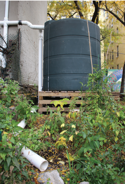
Guiding an overflow pipe into a rain garden.
