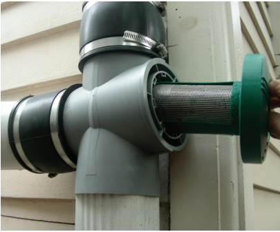
A winterizing tee with a built-in filter.
